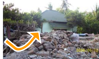
Figure 3 (left) and Figure 4 (right): Two examples of the application of BARRATAGA concept by trained mandors. The two houses have stood completely with very light cracks surrounded by heavy damaged and collapsed regular houses due to the 2006 Yogyakarta-Central Java earthquake
