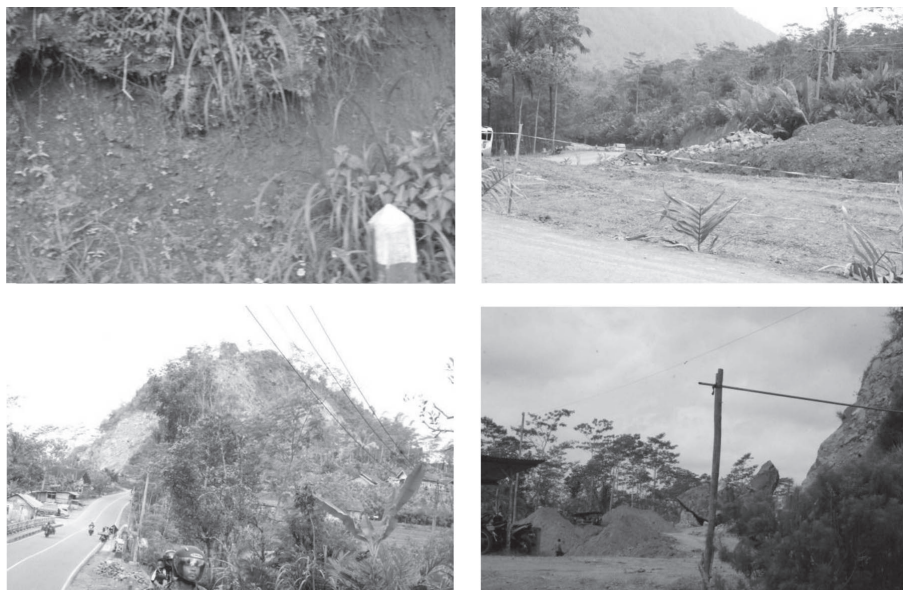
Figure 6. Erosion on open land, May 25, 2017
