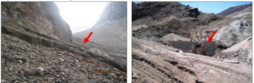
Figure 4.6. Left: inlet tunnel Ganesha, Kanan: inlet tunnel Ampera
