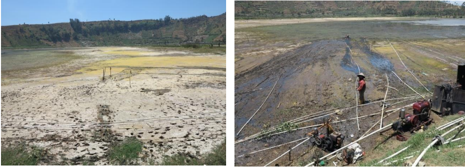
Fig 7. Sedimentation of Merdada Lake, Reducing the Volume
