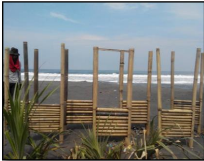
Figure 10. The condition of Apo-apo is still good and strong
