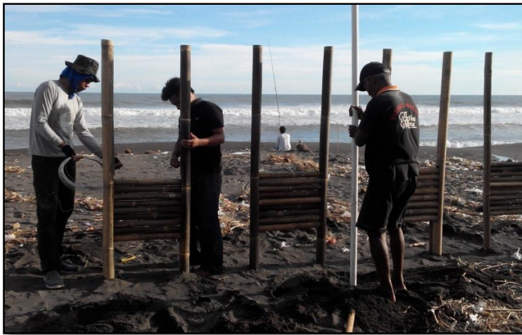
Figure 3. Installation of Apo-apo
