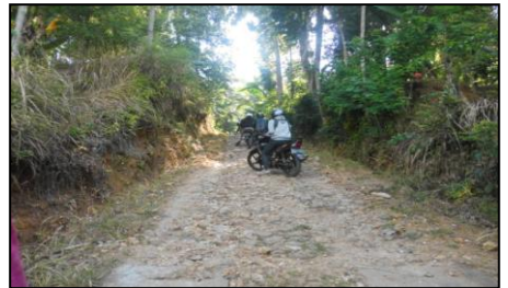
One of Infrastructure of Sidoasri
