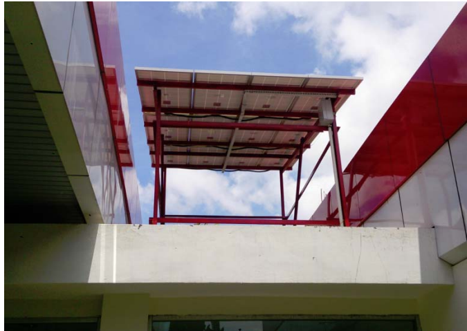
Figure 6. Solar panel installation
