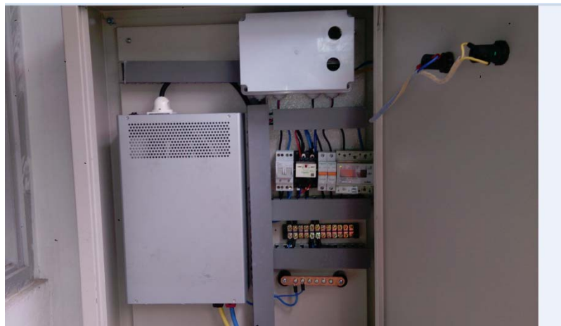
Figure 8. Inverter and hybrid controller panel installation
