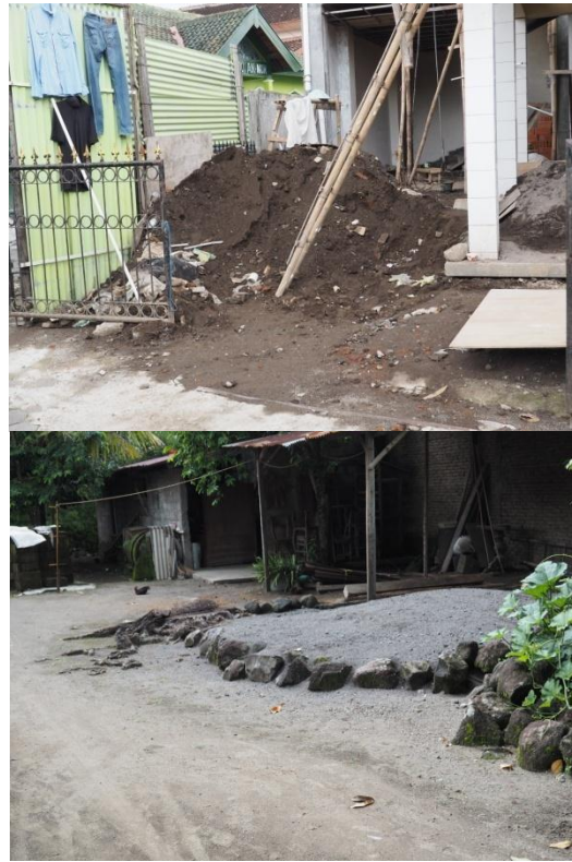
Figure 7. Construction of Houses Leaving Materials Stacked on Road Side
