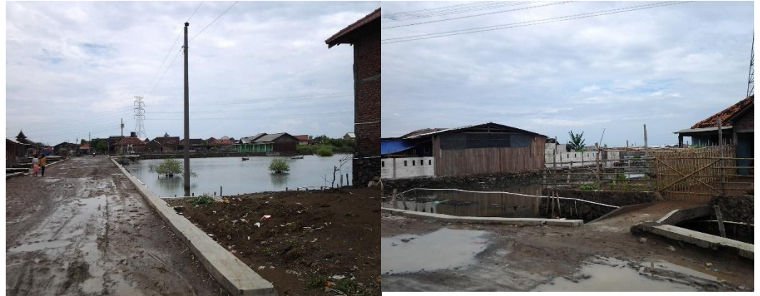
a. Making Road Embankment
