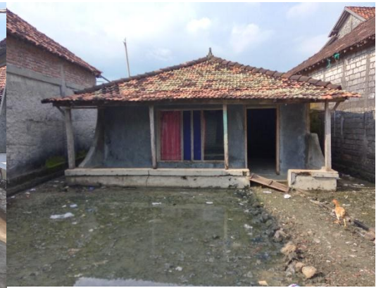
d. Making Embankment in front of House
