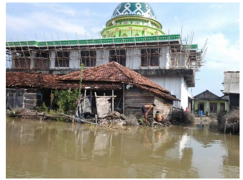
b. Settlements and public facilities flooded
